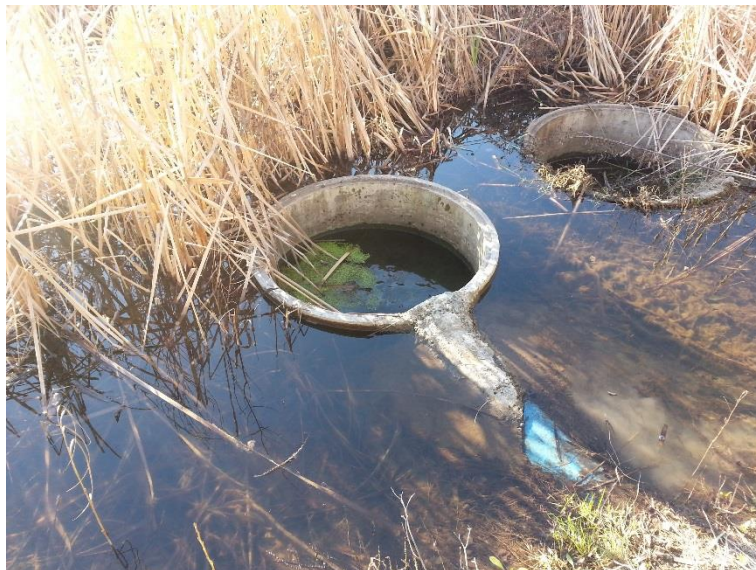
Figure 2: Culvert upstands within stormwater pond
